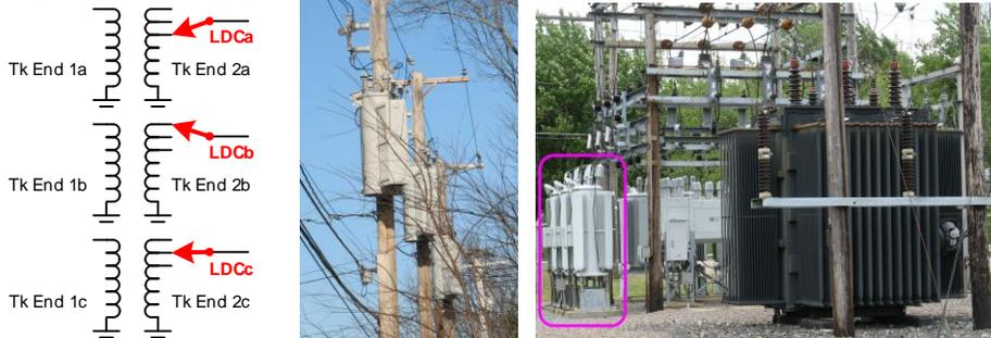
Figure 9: Independent Single-phase Tap Changers apply to CIM TransformerTanks on a Feeder (center) or in a Substation (right). Three-phase examples are shown here, but single-phase and two-phase open-delta configurations also appear on real feeders.
